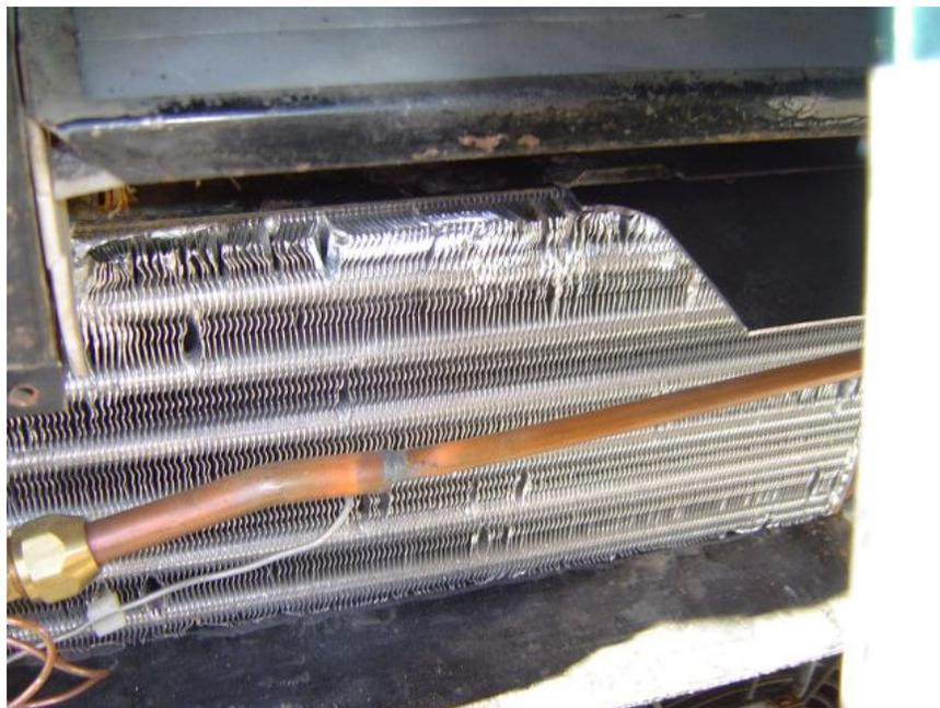
The top of that black plastic diverter is also even with the top of the evaporator. The diverter is a register deflector from Home Depot. It is adjustable to accommodate different size floor registers but even at its shortest, it was too long so I sawed off some of it until it was the right length for the blower case and pop riveted it in place and caulked all seams.
