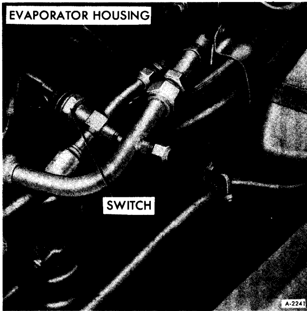
Figure 17—Low-Pressure Cut-Off Switch
