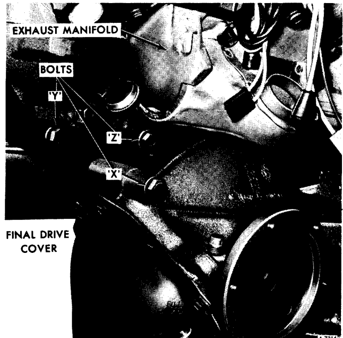
Figure 1—Disconnecting Final Drive From Engine
