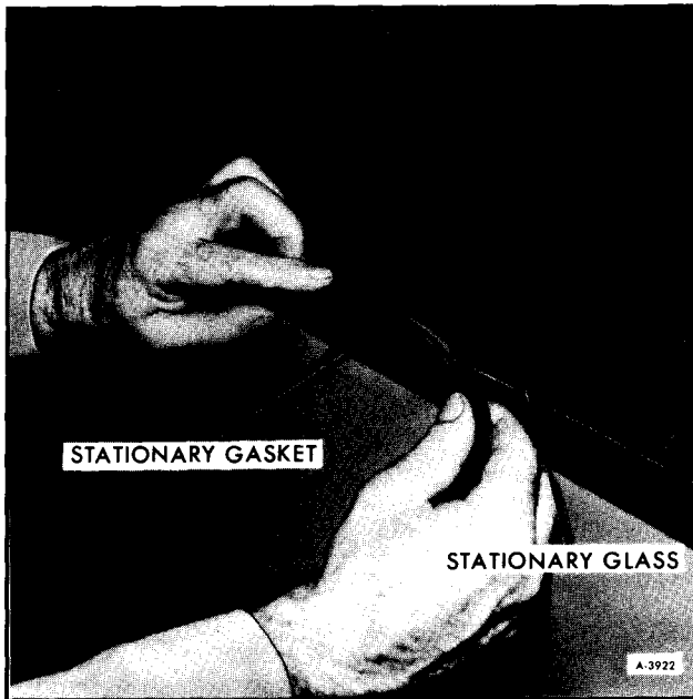
Figure 18—Installing Stationary Gasket
