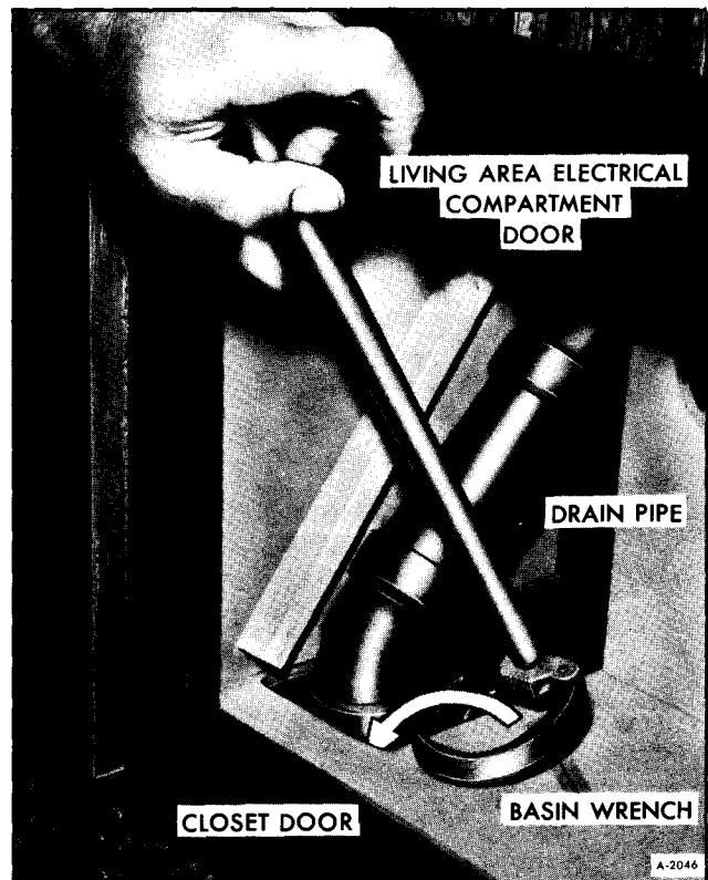
Figure 3—Loosening Pipe Fitting
