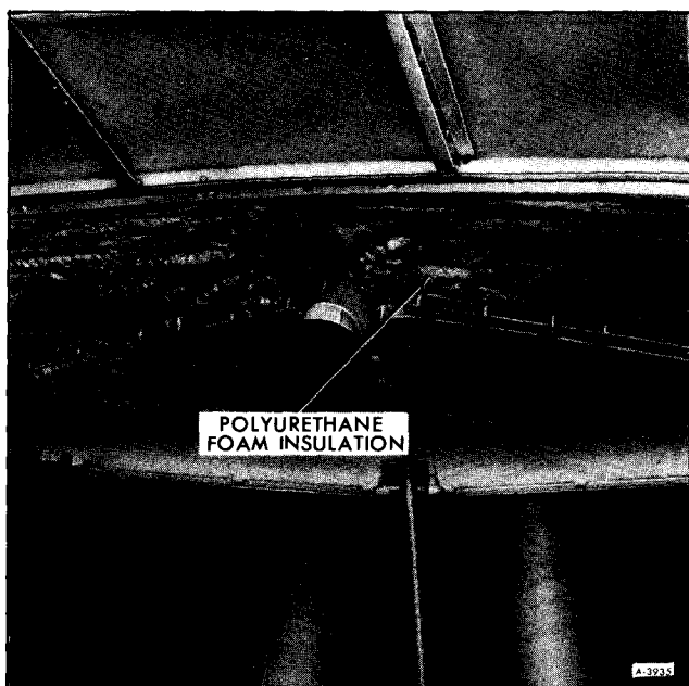
Figure 37—Cab Roof Insulation
