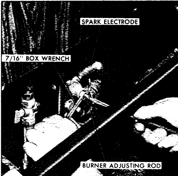
Furnace Primary Air Adjustment
