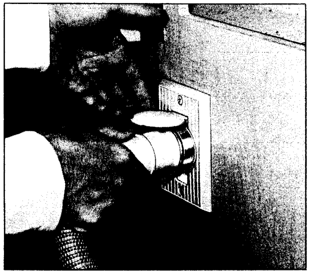
Connecting Flex Hose to Wall Socket
