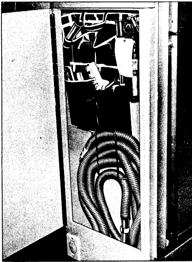
Vacuum Cleaner Components (Typical)
