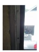
Across the top and bottom are 1/2x 12-14" strips with three screws each. Some of these screws did NOT want to come out and a couple had to be drilled out.
