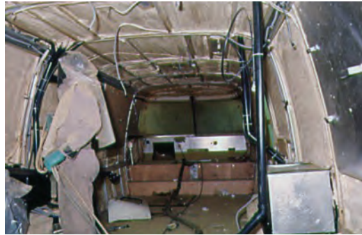
Spraying of foam insulation.
